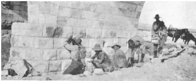
PLACING THE CHARGES.
