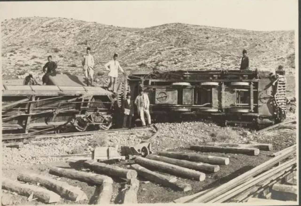
Railway Accident at Wady Sarar.
