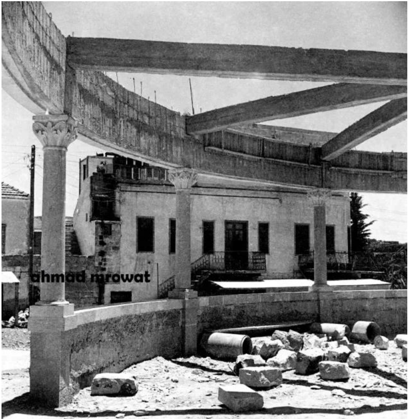
The Jarjoura café building in Nazareth under construction, July 1935. From the Nazareth page gallery on Palestinina.
